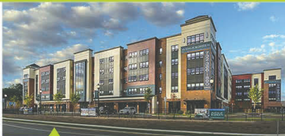
AVENUE & GREEN | WOODBRIDGE, NJ
